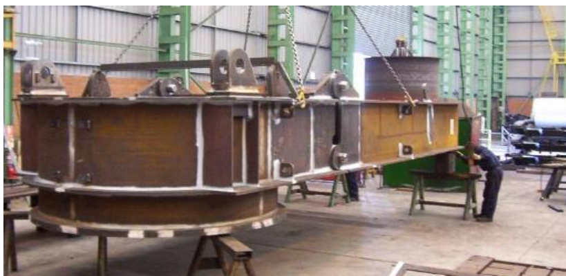
Offshore Crane Welding to AWS D1.1
